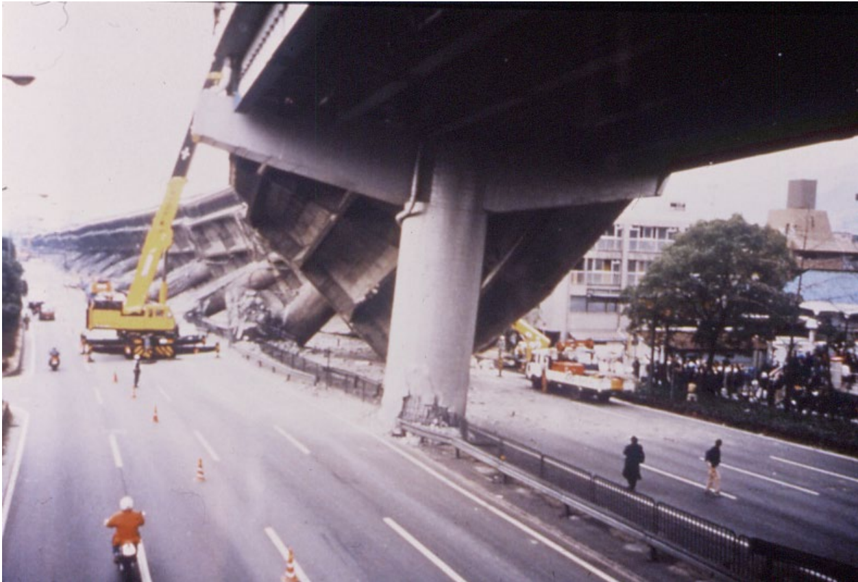
Collapsed Hanshin Highway in Kobe
