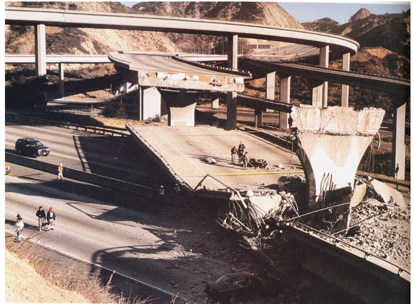
Antelope Valley Overpass after The 1994 Northridge earthquake
