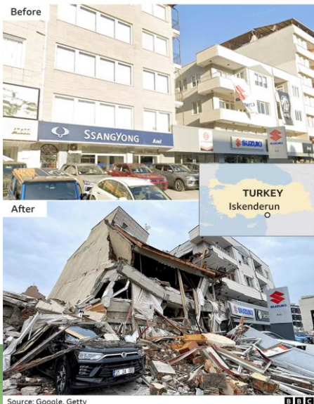
Collapsed building in Iskenderun
