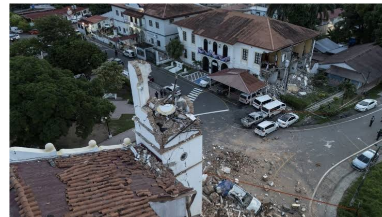
因強地動導致的歷史磚造建物損壞。(圖片來源: Voz.us / 國際新聞網, https://voz.us/en/world/261010/39845/an-earthquake-leaves-at-least-two-people-injured-in-panama-and-causes-several-buildings-to-collapse.html )
